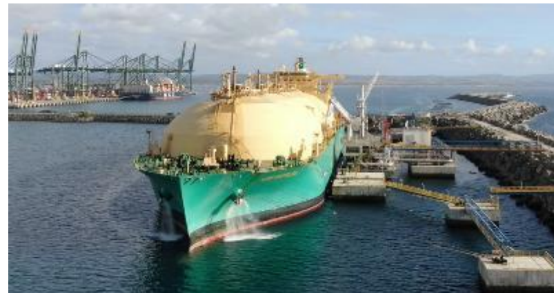
Terminal de Gás Natural
